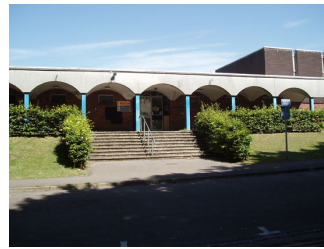
Swimming Pool Building - front
