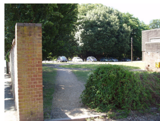
Wyndham Recreation Ground - opening in historic wall
