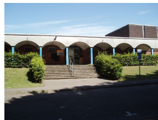
Swimming Pool Building - front
